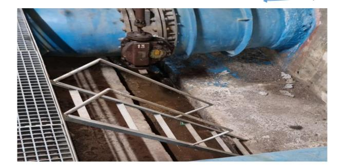
3. Stair Case from Valve operating platform till Mid landing platform. They also need a 600 mm extended across staircase as it would be needed for going across Mid landing platform
