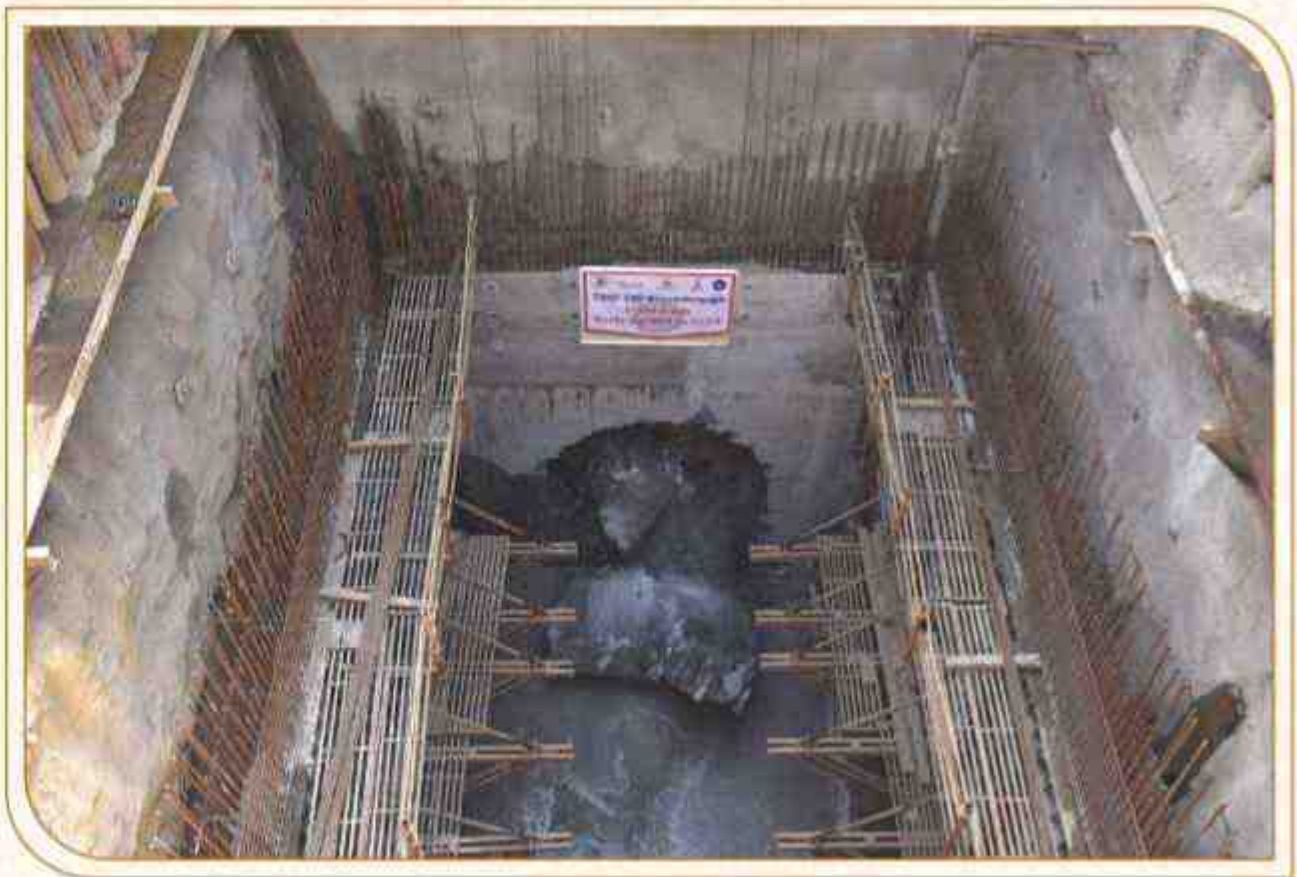
Mithi river tunnel breakthrough
