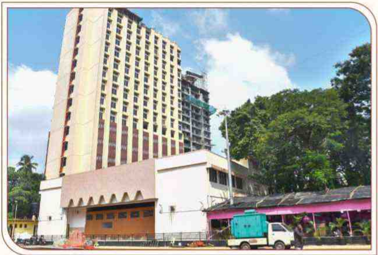
New Building of 'P/East' ward office
