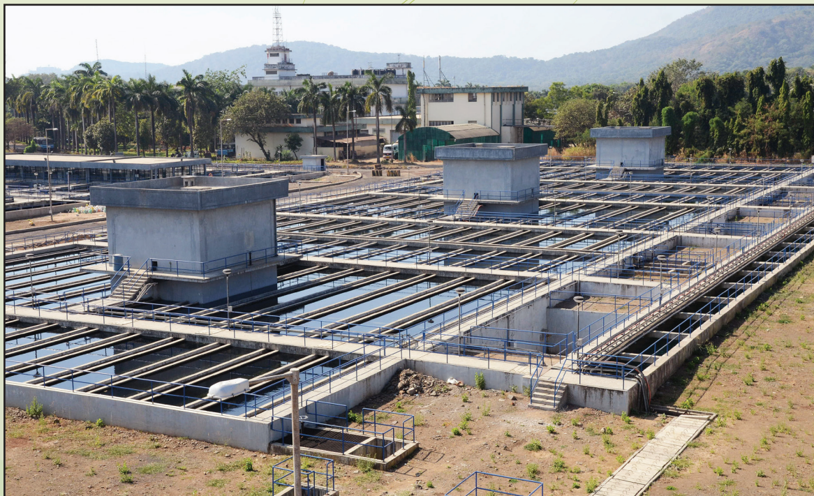
Newly developed filtration plant at Bhandup Complex
